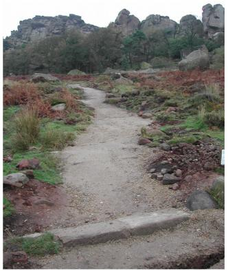
Roaches grit has been crushed into the grit aggregate to help it blend in. The aggregate used for the recent footpath repairs to the diagonal path was obtained from Marchingtons of New Mills; www.marchington-stone.co.uk. The mix was 20 m/m to dust.
